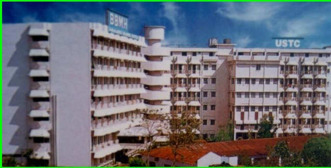
University of Science & Technology Chittagong Main Campus at Chittagong City
